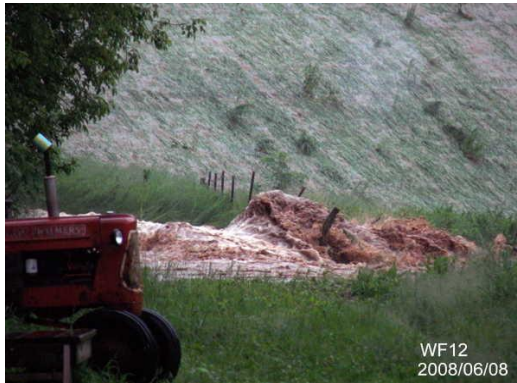
West Fork 12 Overtopping – June 2008
