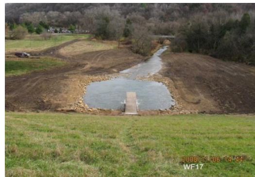
West Fork 17 Stilling Basin Repair – Oct. 2008
