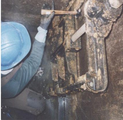
Slide Gate Repair Bad Axe 33
