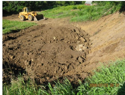
West Fork 12 Aux. Spwy Repair – July 2008
