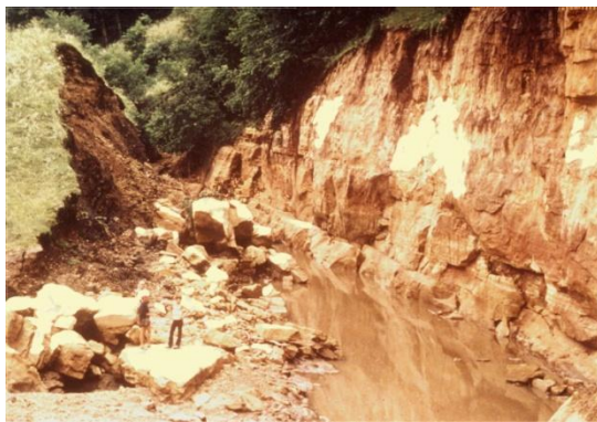
Failure of Coon Creek 41 (Dahlen) 1978
